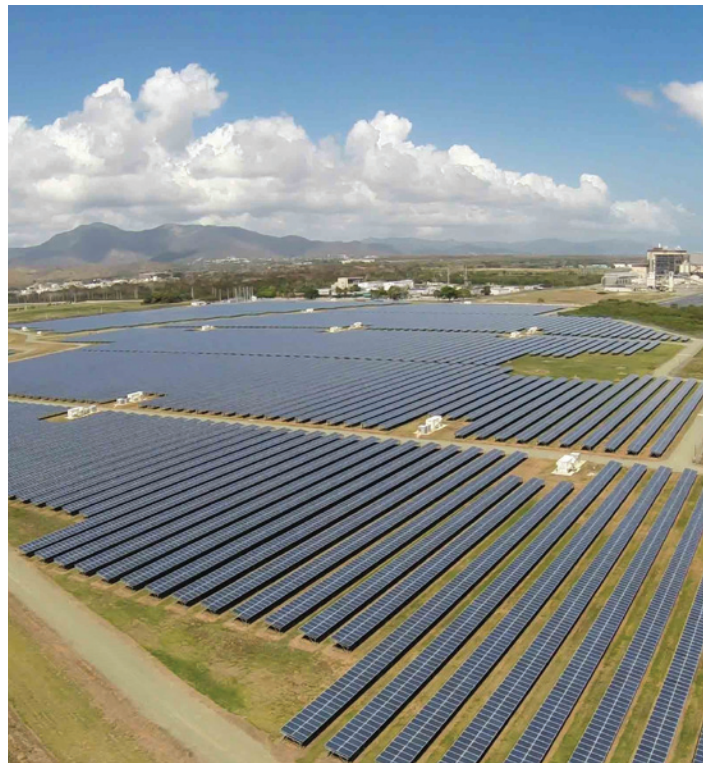
Ilumina, AES' 24 MW solar plant in Puerto Rico.
