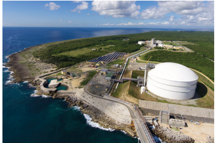
AES Andres LNG Terminal in the Dominican Republic with co-located AES Andres 319 MW CCGT plant and 10 MW energy storage facility.
