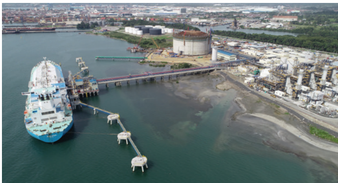
AES Colón 381 MW CCGT plant in Panama co-located with AES Colón LNG terminal.
