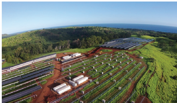
AES Hawaii solar-plus-storage 47 MW of solar photovoltaic capacity and 34 MW of five-hour duration battery-based energy storage project under construction.
