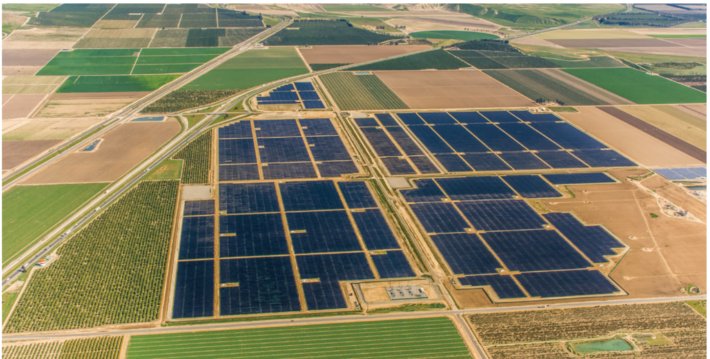
sPower's 72.9 MW Redwood Solar Farm cluster in California.
